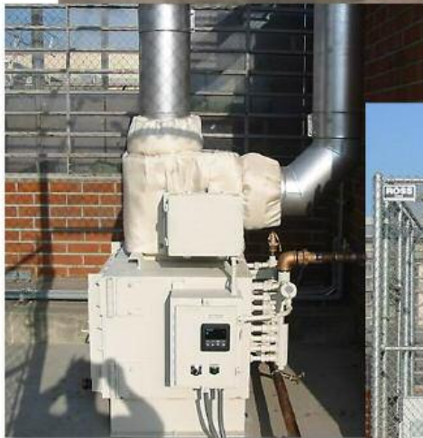
HRSR-116826.5ALS (above) Murrieta High School, Murrieta, California Recovering Exhaust Heat from a natural gas 60kW micro-turbine; cooling 856 SCFM from 580°F to 289°F; and heating 40 GPM of water from 75°F to 90.2°F.
